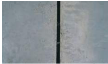
15. Construction joint.
